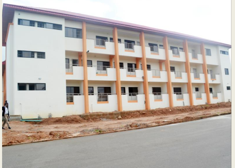
Newly constructed faculty of Basic Medical Sciences, University of Medical Sciences, Ondo located inside the Medical Village, Ondo City, Ondo State
